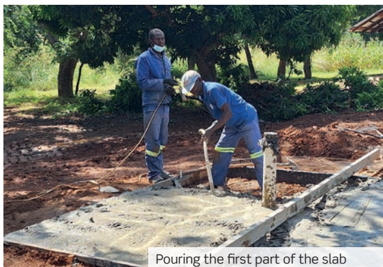
Pouring the first part of the slab
