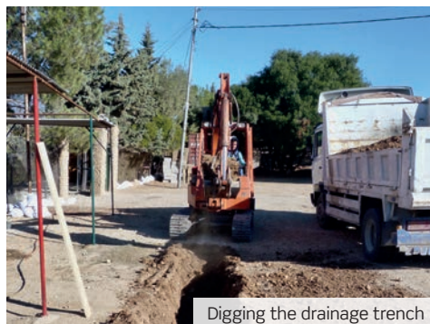
Digging the drainage trench
