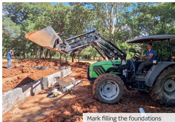
Mark filling the foundations
