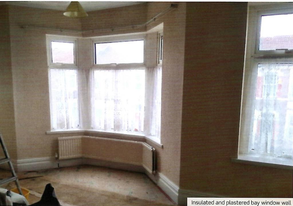
Insulated and plastered bay window wall
